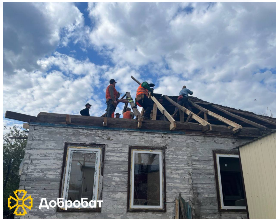
Volunteers working on roof repairs in Hostomel
